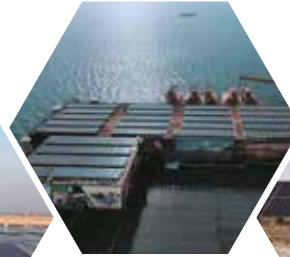
Sea Surface Photovoltaic Power Station, Yantai
