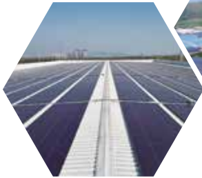
Commercial and Industrial Rooftop Distributed Photovoltaic Power Station, Xuzhou
