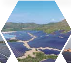
Centralised Photovoltaic Power Station, Sanya
